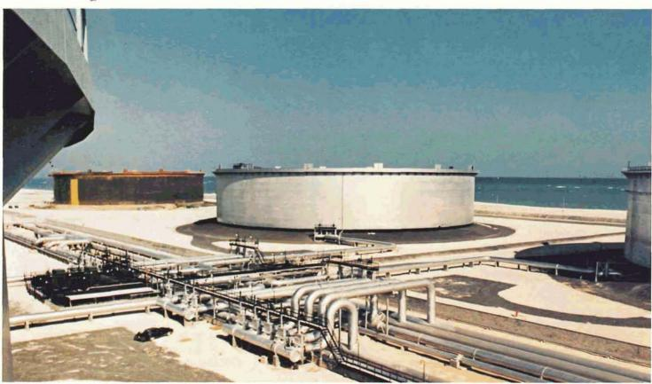
Piping Flexibility A NASA computer program aids Hudson Engineering Corporation, Houston, Texas, in the design and construction of huge petrochemical processing plants like the one shown, which is located at Ju'aymah, Saudi Arabia. The pipes handling the flow of chemicals are subject to a variety of stresses, such
